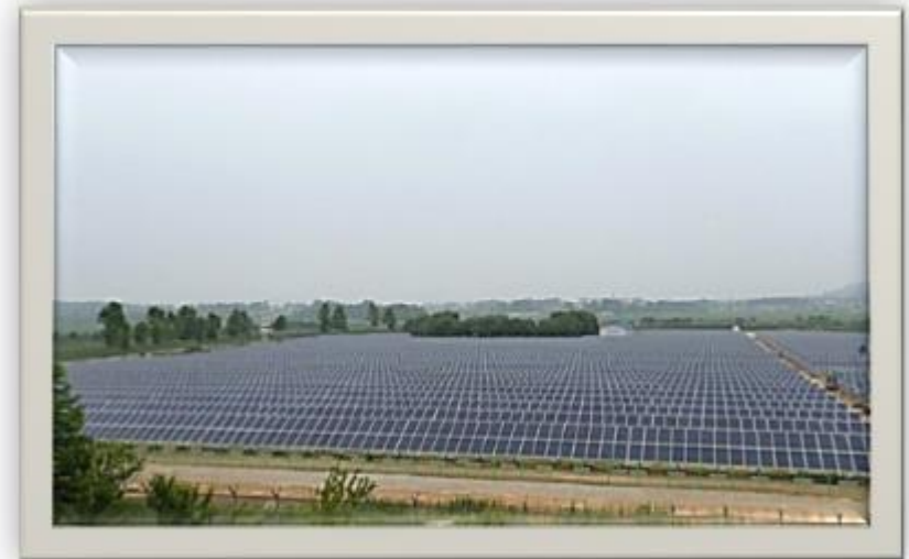
View of Yongsung solar energy(2015)
