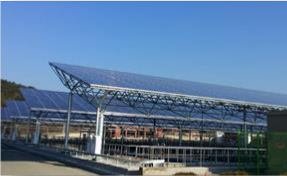
PV for water supply facility (Daegu Solar)
